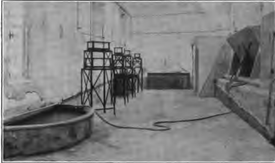
A. SERVICE CORRIDOR OF EXHIBITION AQUARIA WITH FLOOR TANK AND SMALL AQUARIA IN IRON STANDS.
