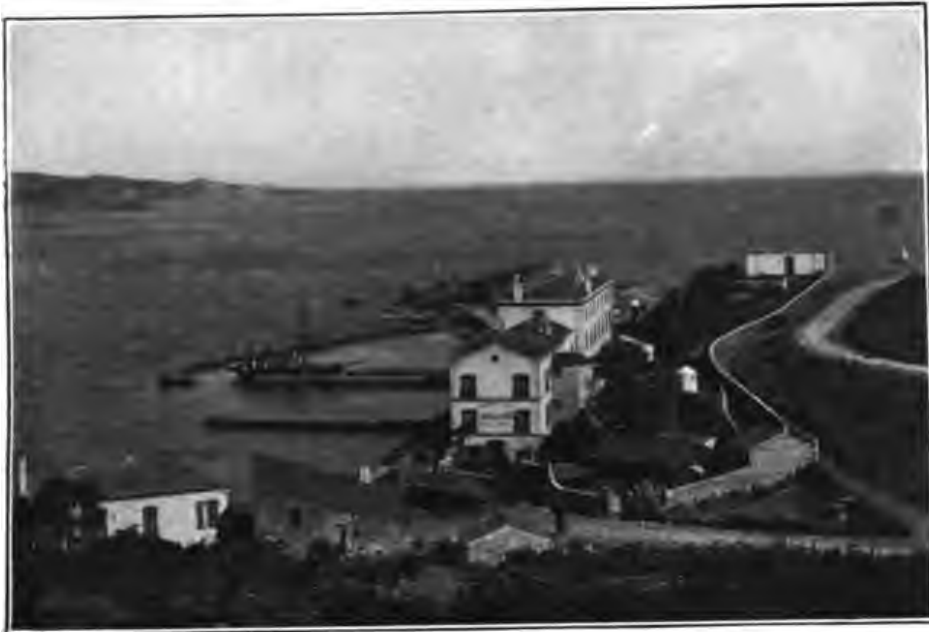
A. GENERAL VIEW FROM THE HILL ABOVE.
