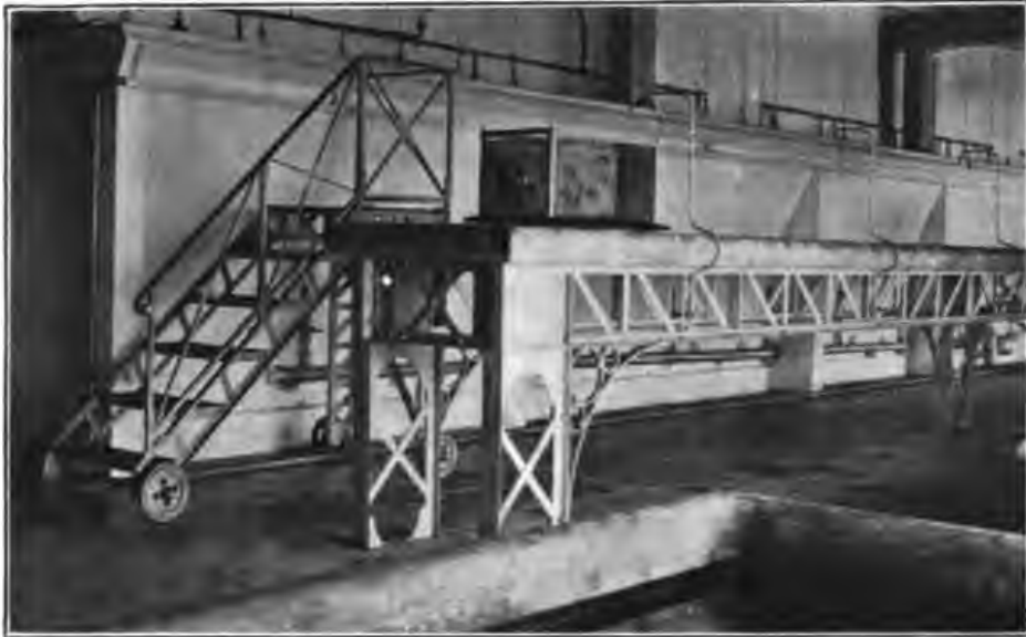
A. REAR OF EXHIBITION AQUARIA, ROLLING STAIR FOR ATTENDANCE, AND RACK FOR EXPERIMENTAL AQUARIA.
