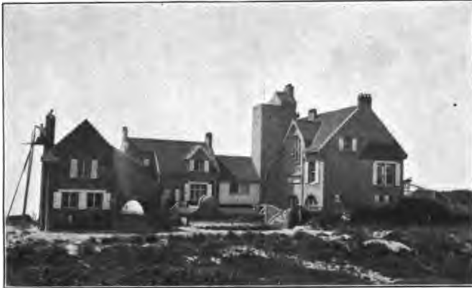
A. STATION BUILDING FROM THE EAST.
