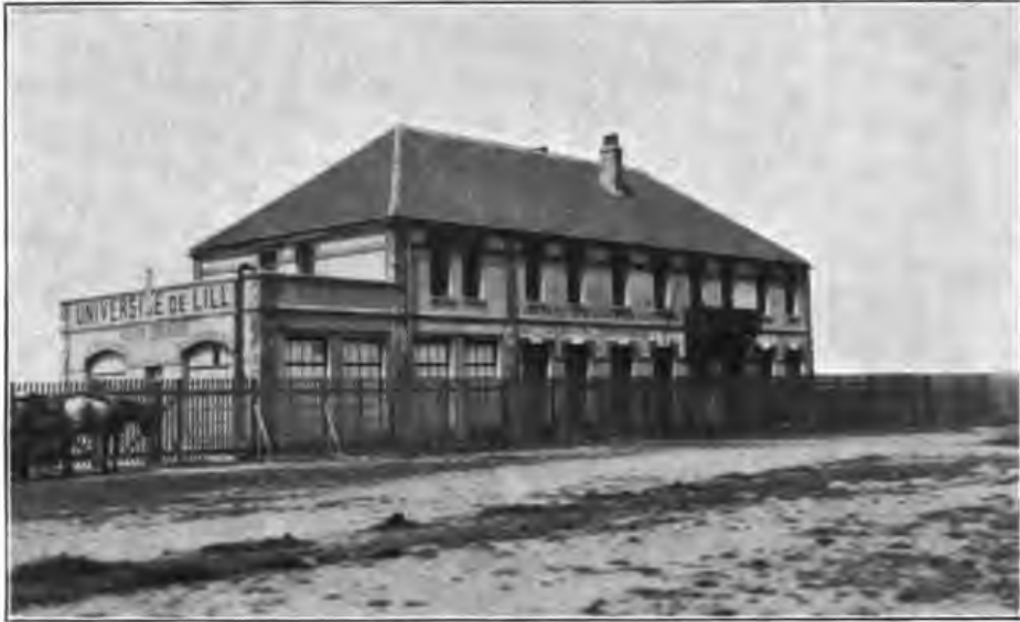
A. STATION BUILDING.
